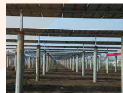
Hebei Shangyi - 21.5MW
